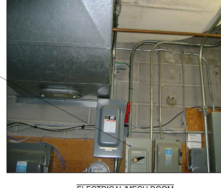
60A DISCONNECT SWITCH TO BE REPLACED WITH 100A DS
